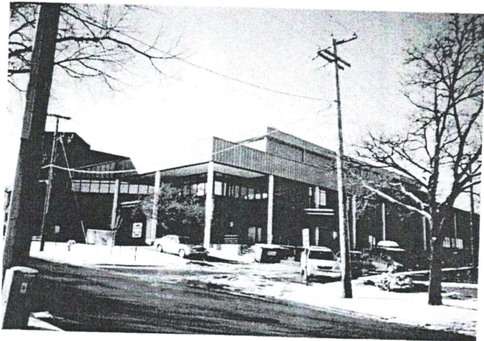
LOOKING IN A SOUTHWESTERLY DIRECTION WITH THE SUBJECT PROPERTY IN BACKGROUND
